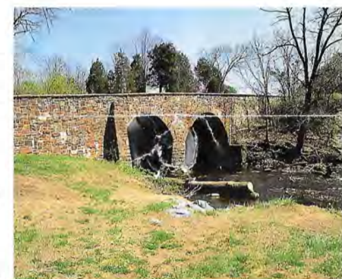
Stone Bridge, tour stop 12
